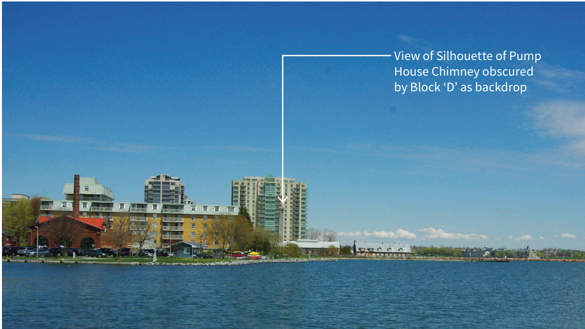
7. Current view north toward the Development Site, from the Kingston Yacht Club (Source: IBI)
