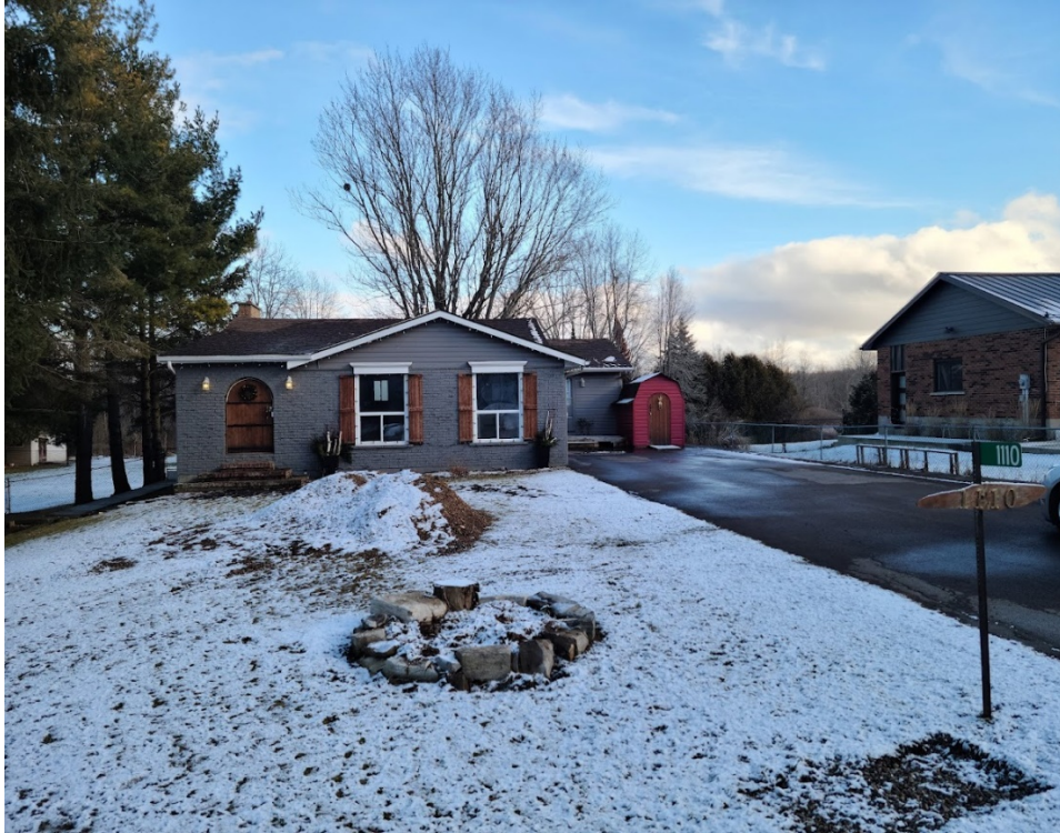
Figure 1: Frontal view of the subject property at 1110 Westbrook Road.
