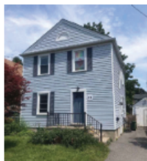
EXISTING FRONT ELEVATION IMAGE
