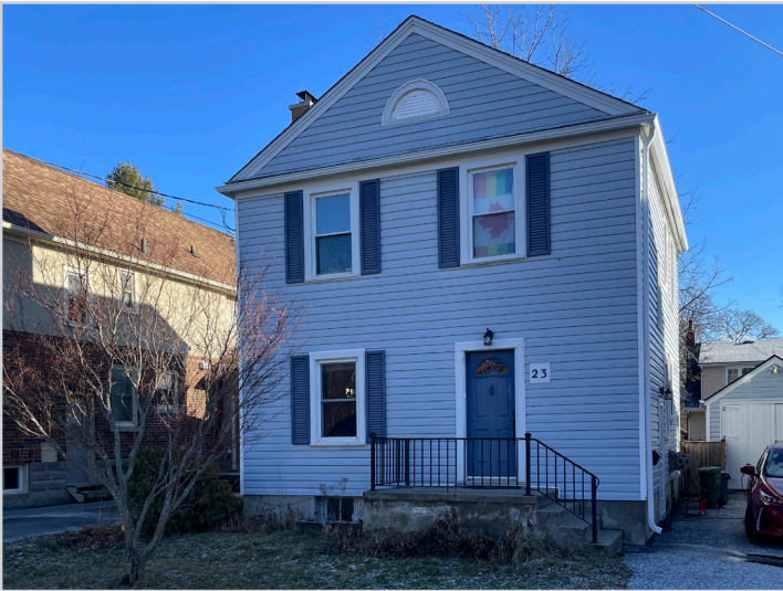
Figure 1: Looking east at the front of the subject property.
