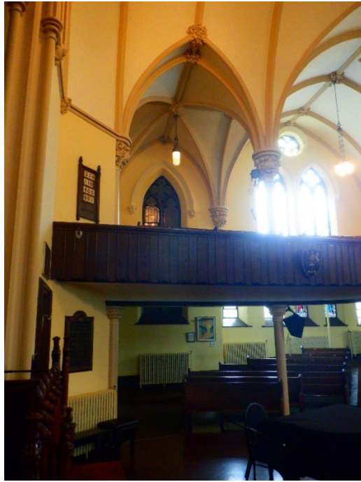
Figures 22 & 23: Pointed arch intersecting side vaults with plaster ribs and decorative bosses. (Heritage Studio, June 2023)
