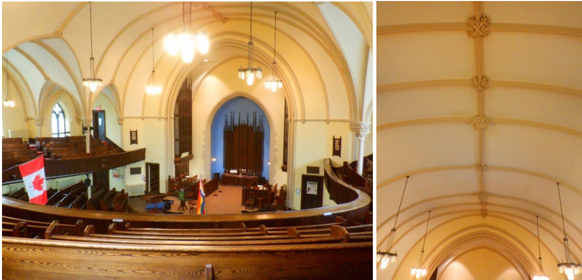
Figures 26 & 27: Looking down towards the pulpit from the gallery, barrel-vaulted main ceiling, and moulded plaster ribs and decorative bosses. (Heritage Studio, 2023)
