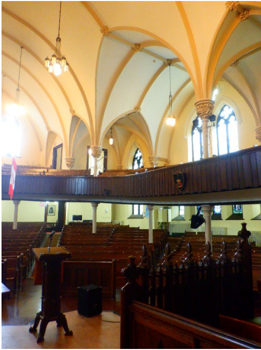
Figures 22 & 23: Pointed arch intersecting side vaults with plaster ribs and decorative bosses. (Heritage Studio, June 2023)
