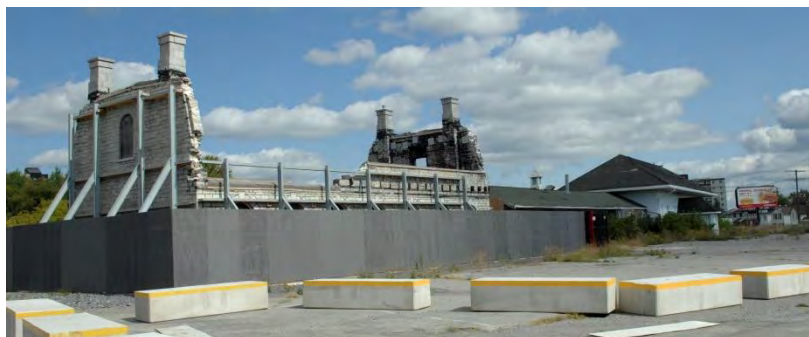
2011 with the roof and interior fittings removed
