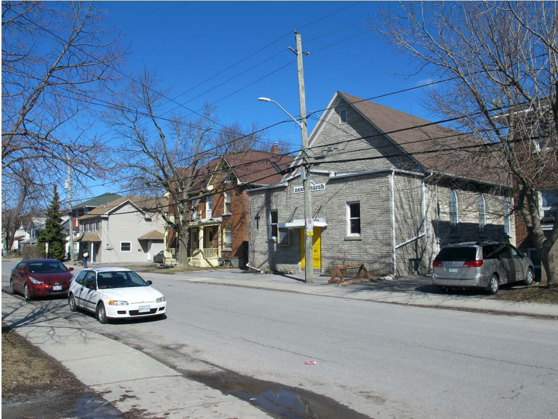
Converted church on Colborne Street
