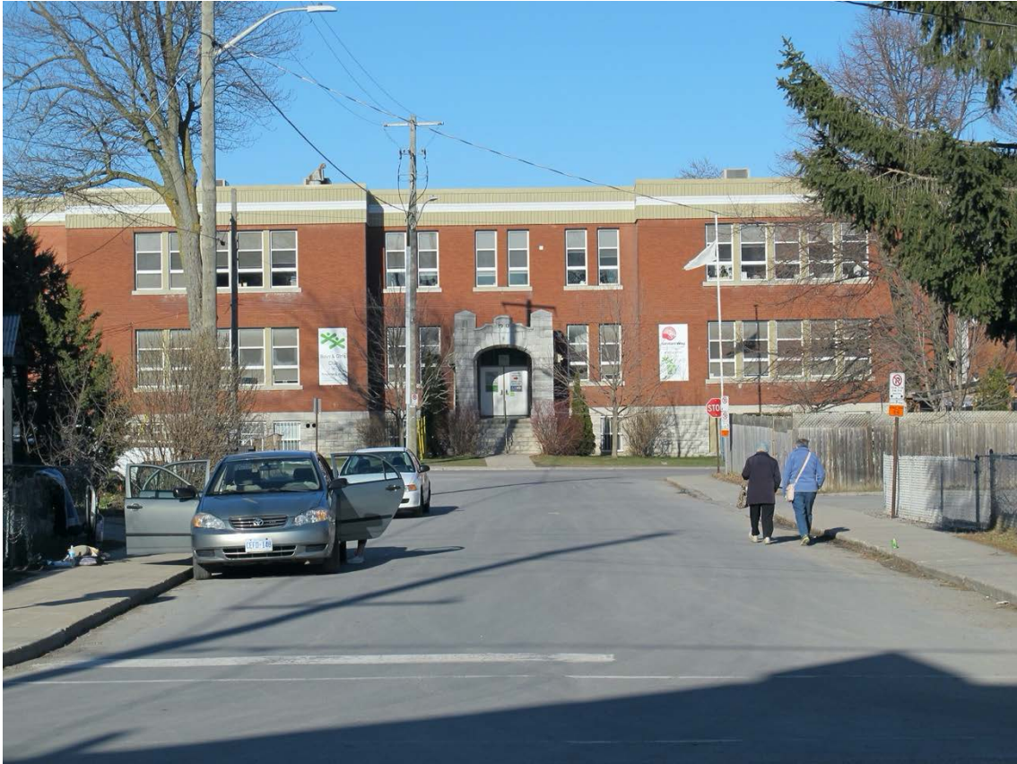
Converted school on Bagot Street
