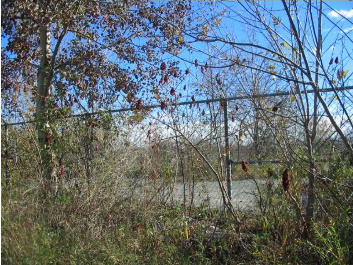
Foundations of former tile works
