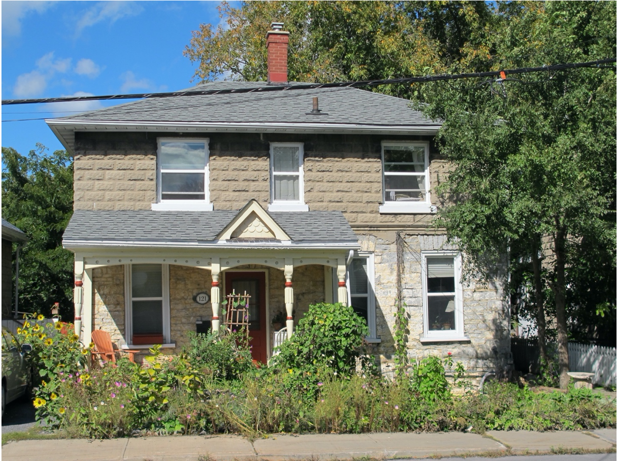
Rehabilitated house on Raglan Road
