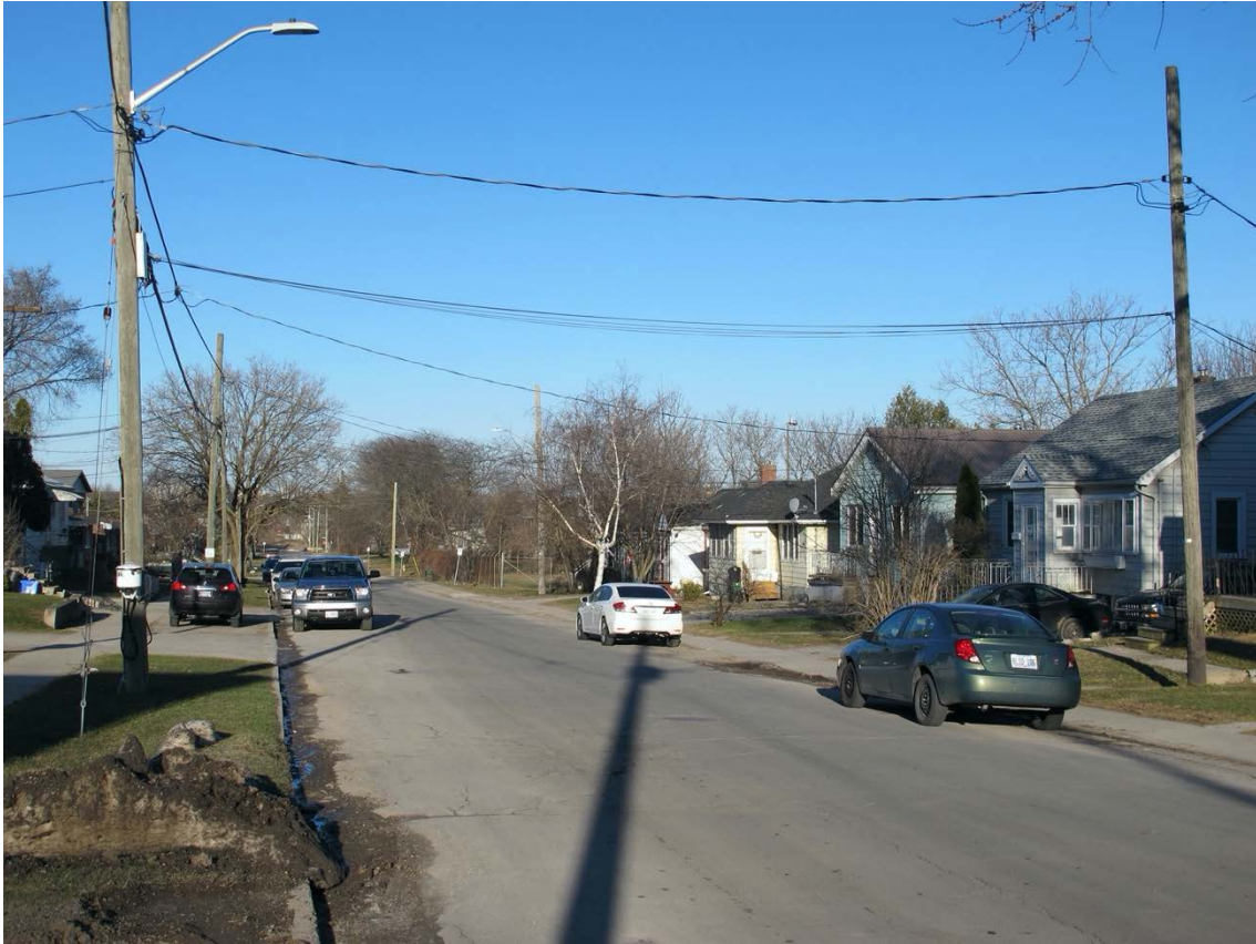
Long residential block on Fraser Street
