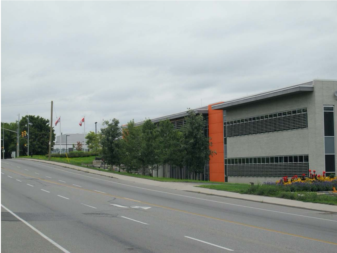
City of Kingston buildings at Barbara Avenue
