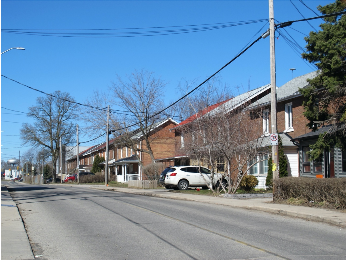
Row of semi-detached housing on Stephen Street
