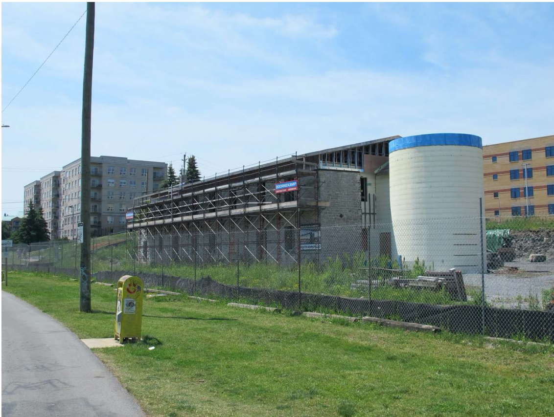
Former oil storage building
