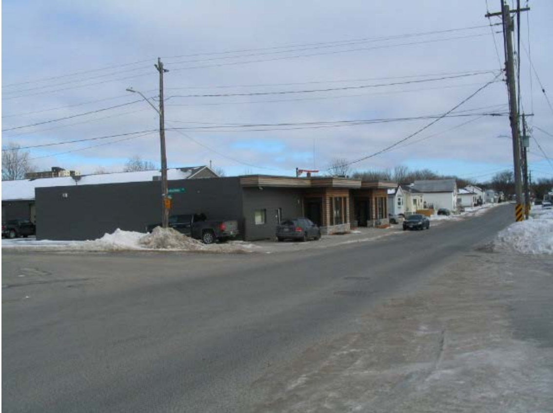
Industrial/commercial buildings on Hickson Avenue
