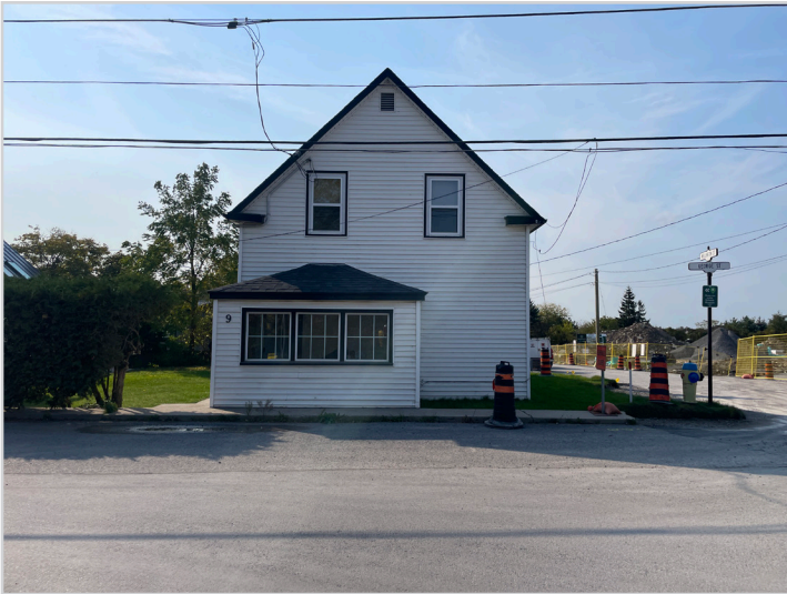
Figure 1: Looking west at the front of the subject property.
