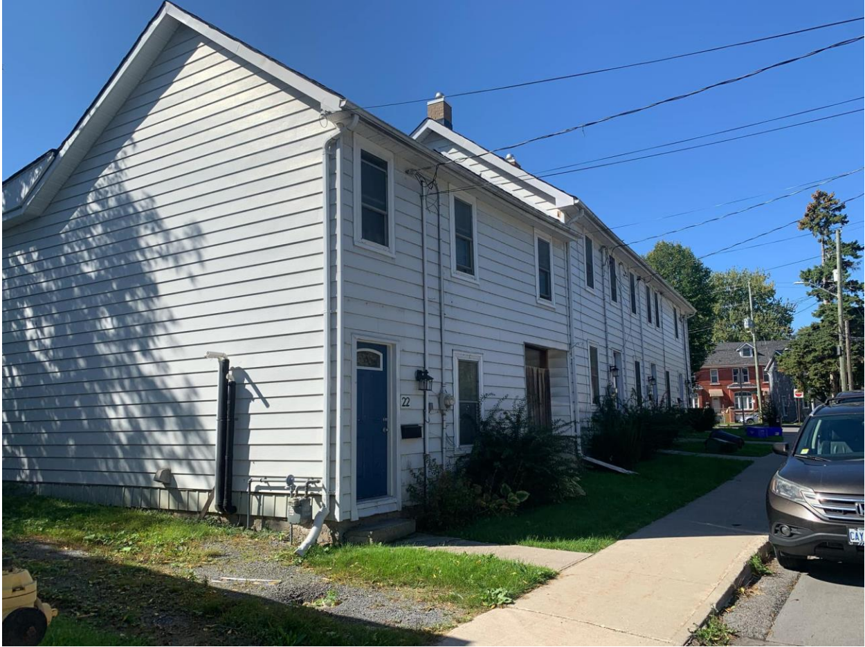
Figure 2: Existing sidewalk and walkways located along the front of the subject property along the Ellice Street frontage (September 26, 2024).
