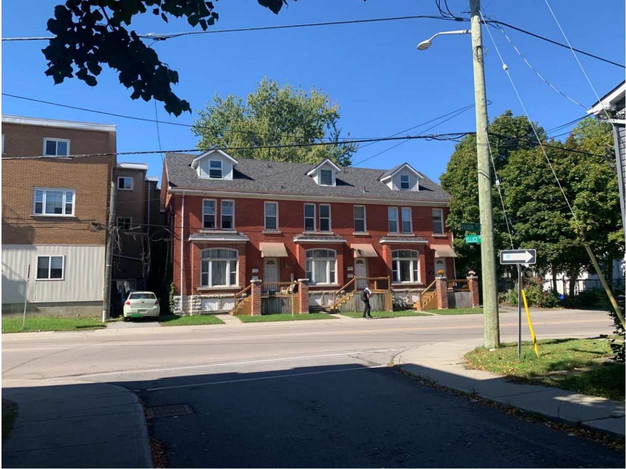
Figure 10: Existing built form in the surrounding area, properties addressed as 228-232 Division Street (September 26, 2024).
