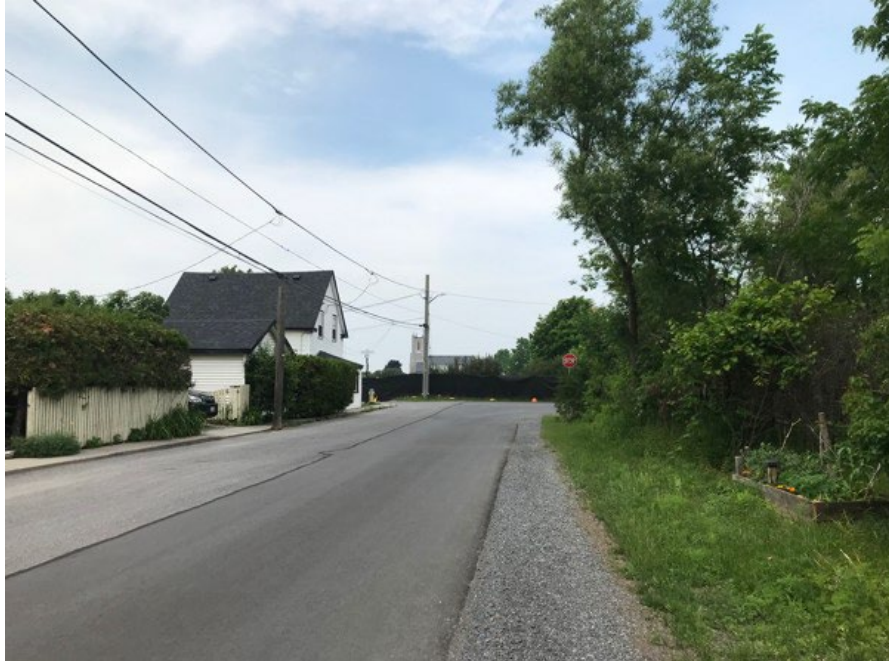
Figure 10: Looking north along George Street, toward the subject property and St Marks Church, June 2024.
