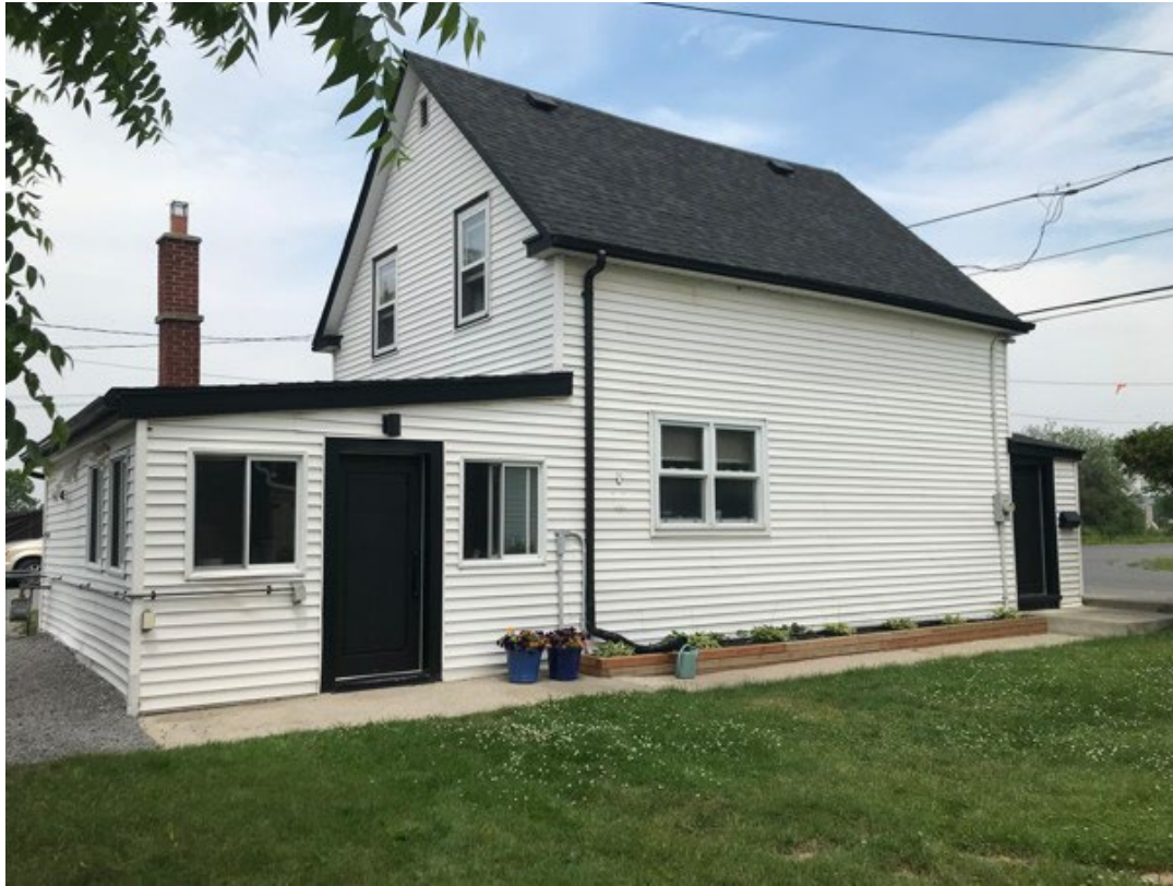
Figure 16: South elevation showing two existing contemporary entrances.
