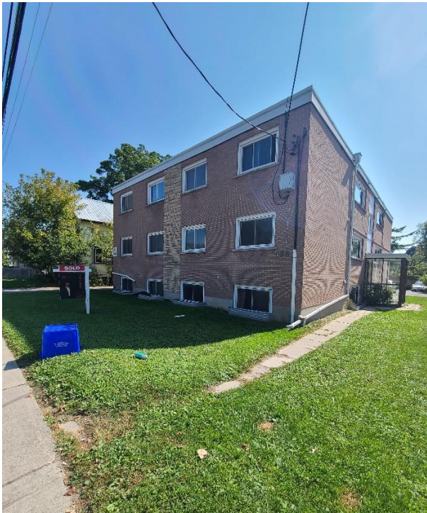
Figure 1- Front of building from Concession Street
