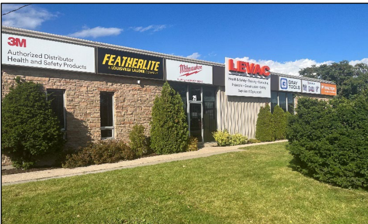
Figure 2: Photo of 25 Railway Street principal building frontage
