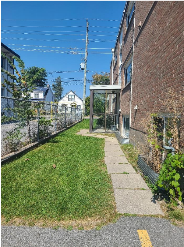
Figure 2- Existing walkway from rear parking lot. To be expanded to 1.1 metres from existing width.
