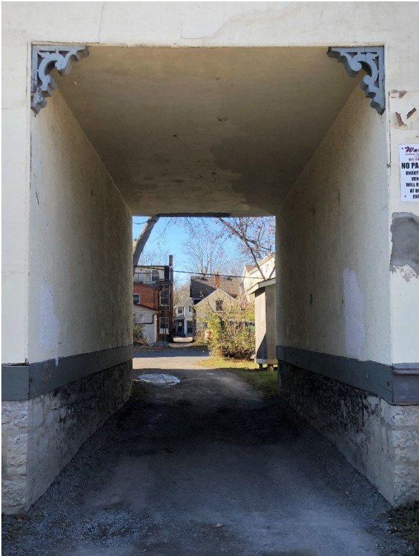
Figure 2: View through carriage way to backyard.
