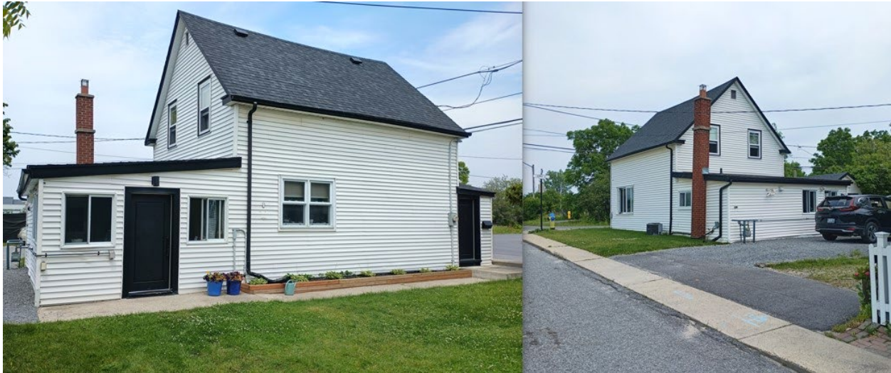
Figure 3: South elevation (left) and west elevation (right), June 2024.
