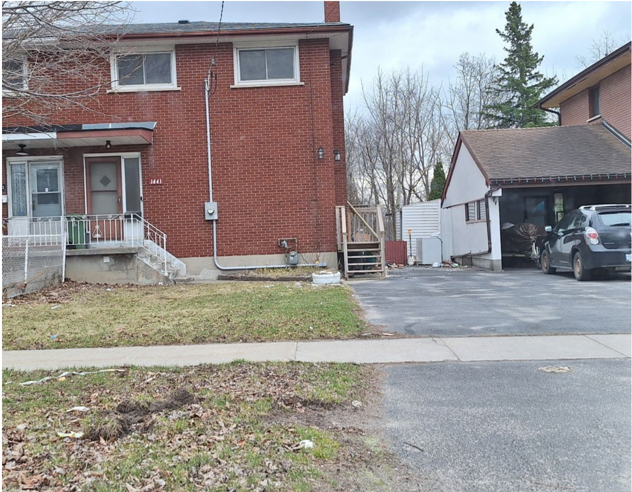
Site Photo – 1441 Montreal Street
