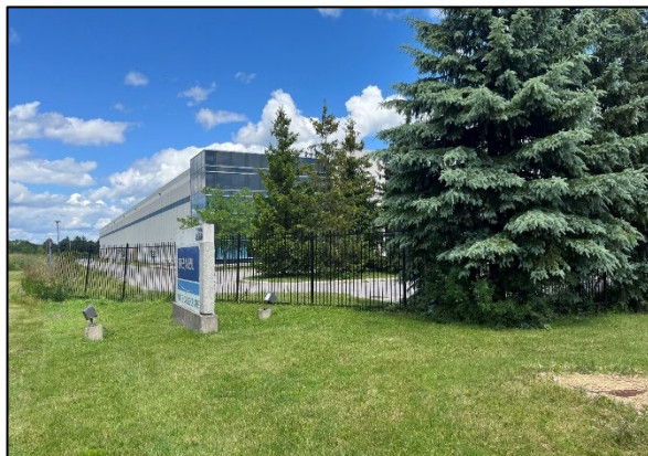
Figure 6: View of east side yard from Innovation Drive.
