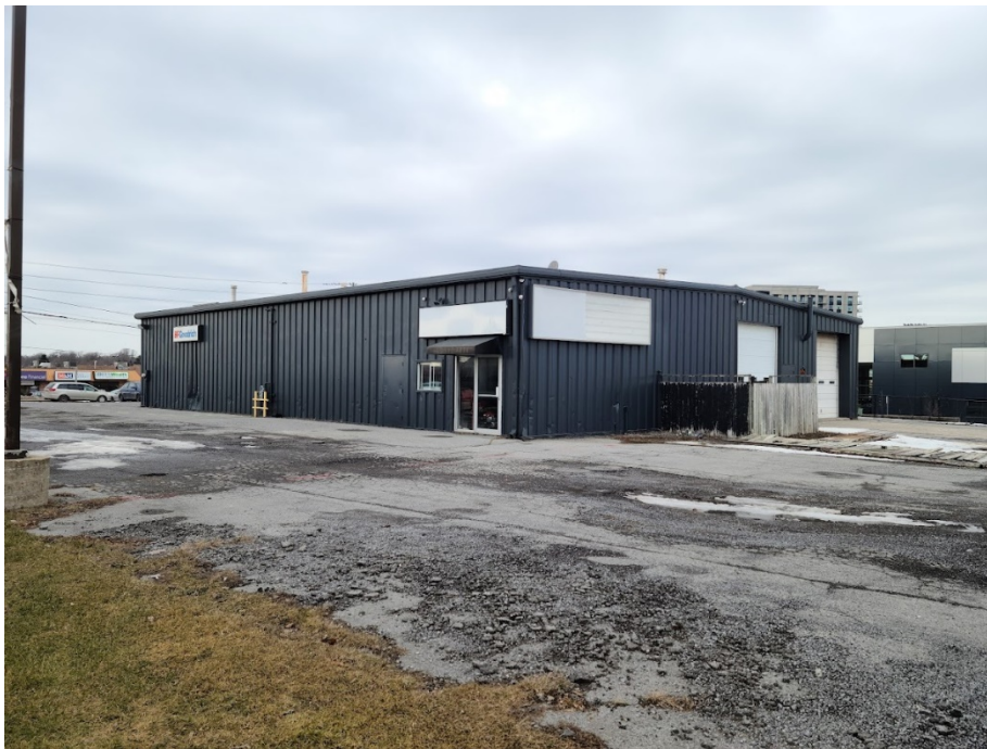
Figure 2: View of the rear and side of the existing vacant building from the sidewalk adjacent to Taylor-Kidd Boulevard. Existing building will be demolished before the construction of the new car wash.
