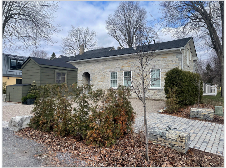
Figure 2: Looking northwest at the shed adjacent to the existing accessory structure to the north.
