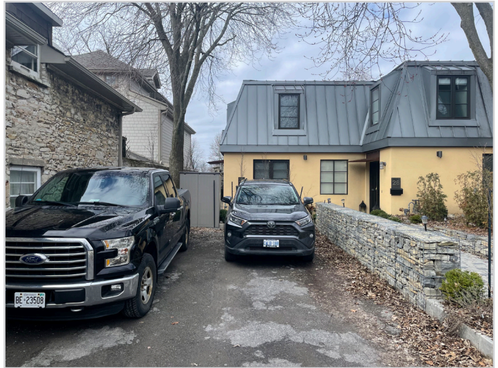
Figure 2: Looking west at the structure in front of the semi-detached home.
