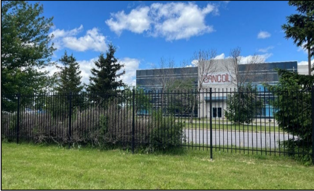
Figure 1: View of 933 Innovation Drive from the street frontage.
