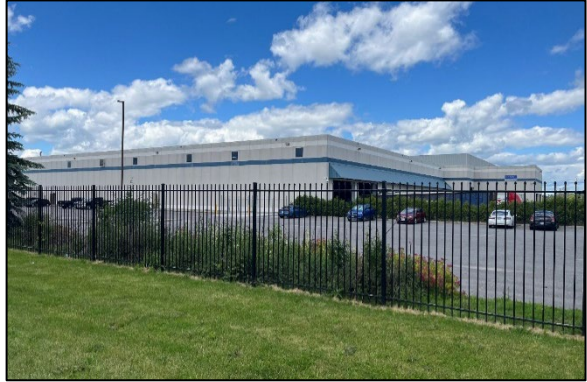
Figure 2: View of eastern extent of existing building from the street frontage.
