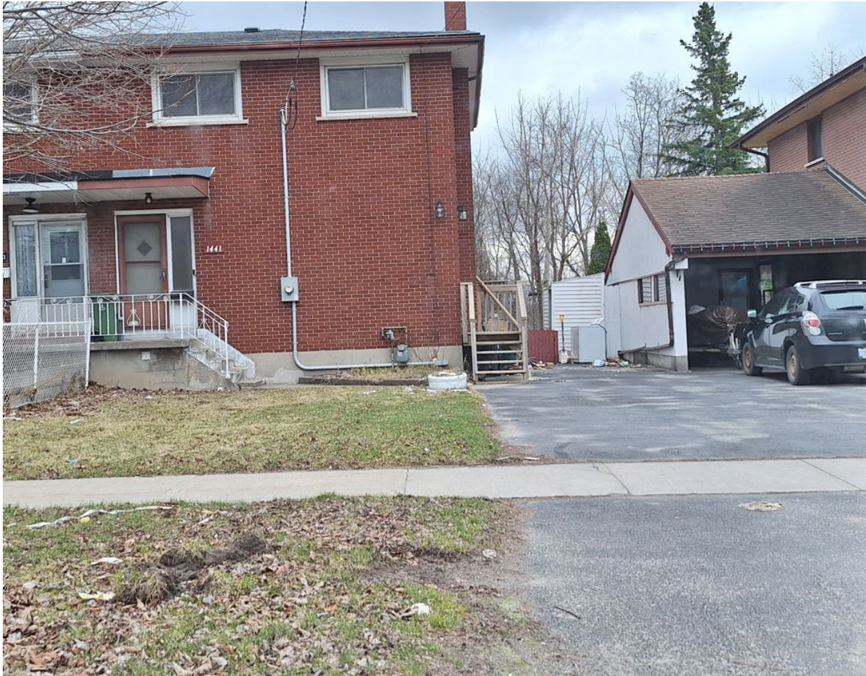
Site Photo – 1441 Montreal Street
