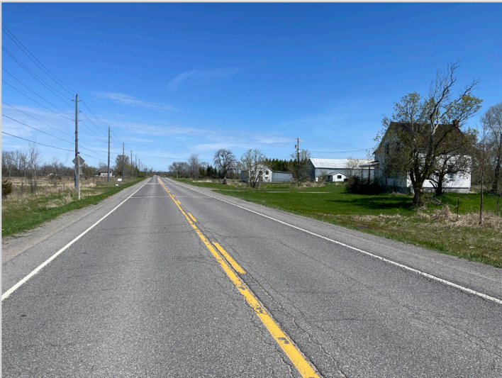
Figure 3: Looking east at the dwelling and farm buildings on the subject property on Unity Road.
