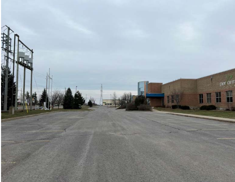
Figure 3: Parking area at the front of 1287 Gardiners Road.
