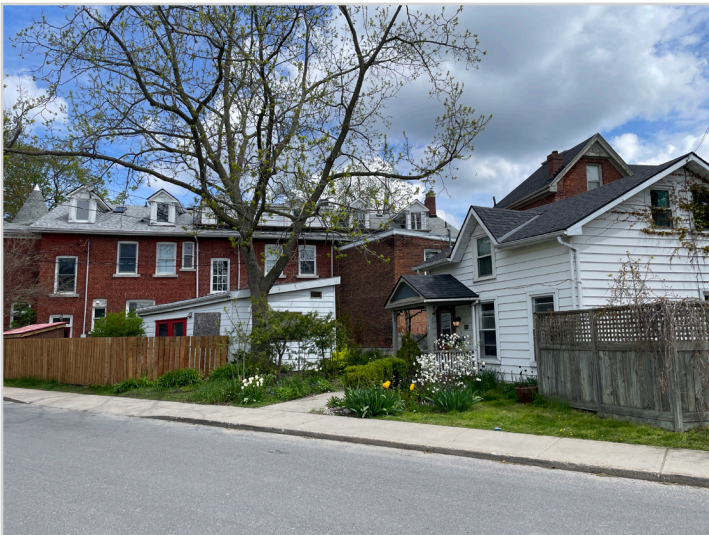
Looking northeast along West Street at the rear of the subject property.
