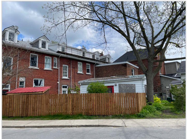
Looking northeast along West Street at the rear of the subject property.
