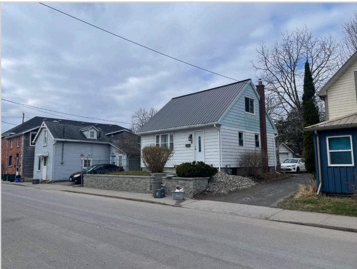
Looking southwest along Cowdy Street past the subject property.
