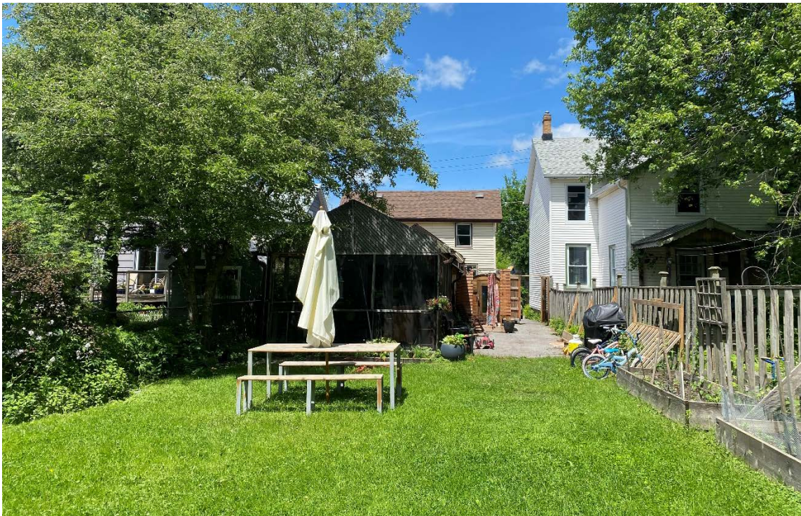
Figure 2: North facing view of the existing house from the rear yard.
