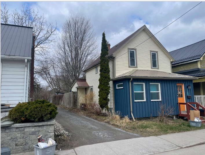
Looking northwest at the subject property and the existing addition in the rear yard.
