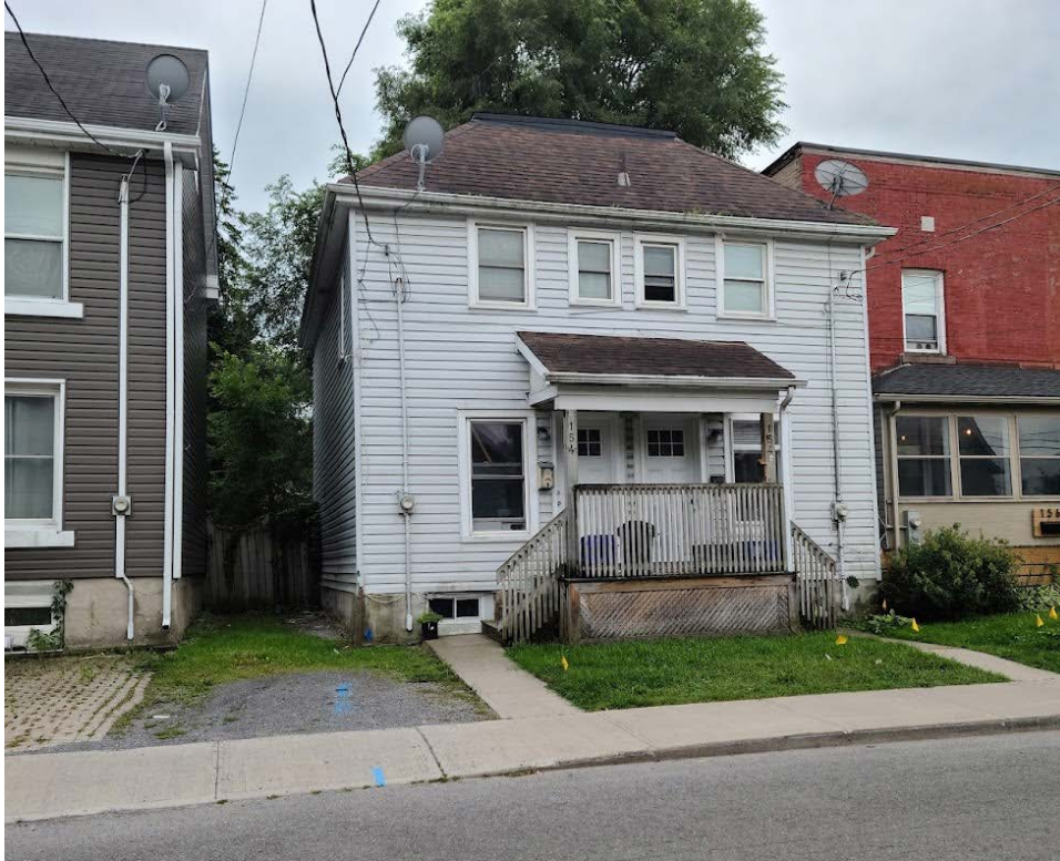
Figure 1: Frontal view of the semi-detached dwelling at 154 Pine Street.
