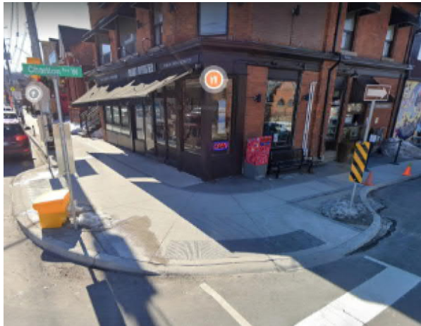
Curb Bump Out
