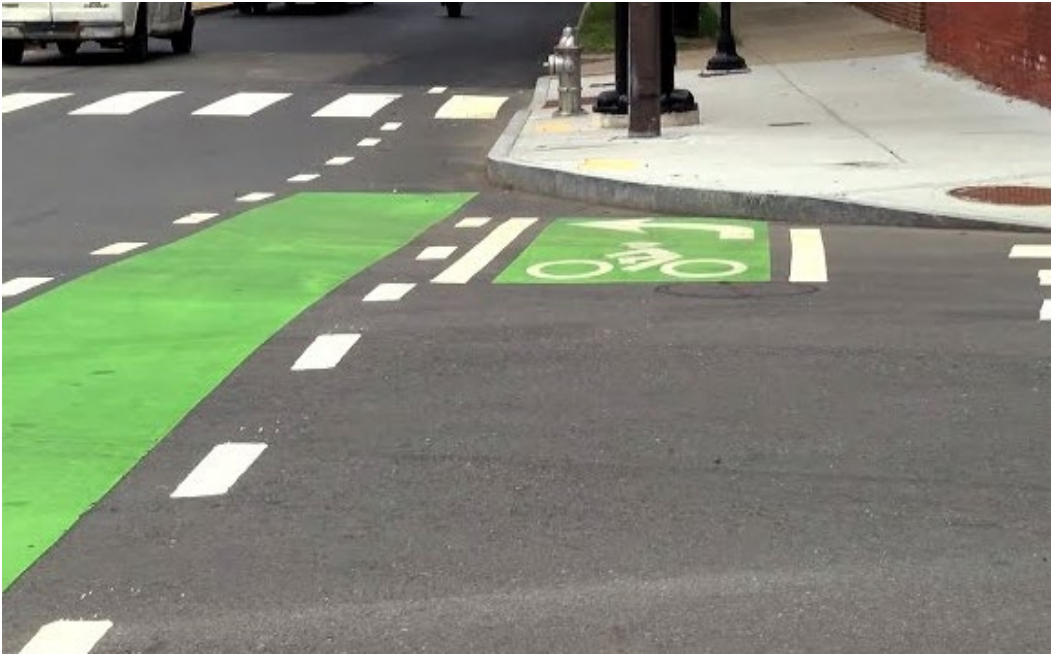
Figure 3: In-Lane Two-Stage Bike Turn Box
