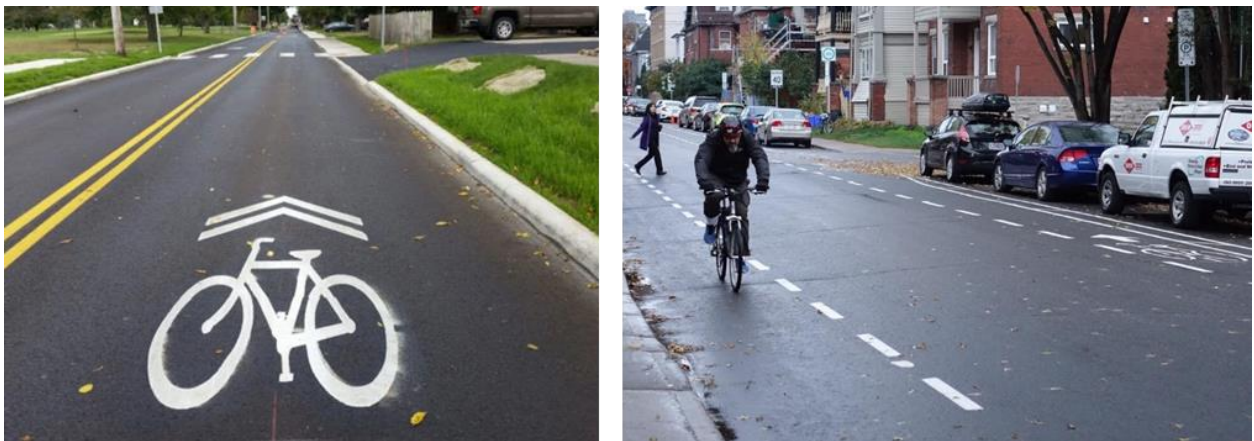
Sharrow pavement marking in London, ON Advisory bike lane, Ottawa, ON
