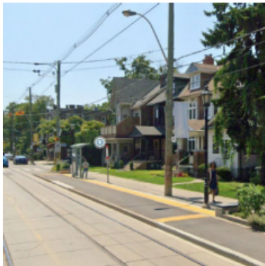
Cycle track raised to sidewalk height at transit stop, Toronto, Ontario (Source: Google Maps) Cycle Track Separated by
