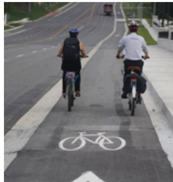
Mountable Curb, East Gwillimbury, Ontario (Source: OTM Book 18 Cycling Facilities ) Raised cycle track on Bloor
