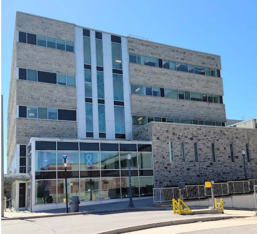
Figure 5: Kinesiology and Health Studies building at 28 Division Street. View from west side of Division Street. Kinesiology and Health Studies building is proposed to be rezoned to IN2. No Exception Overlay is proposed for this building.
