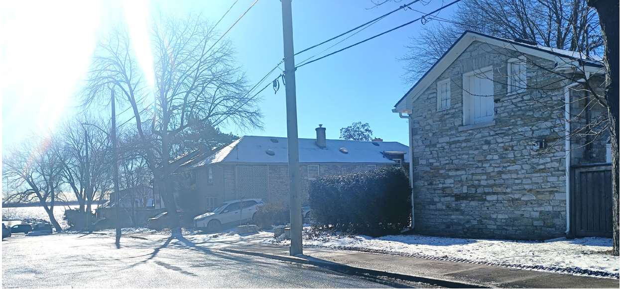
Figure 7: Maitland Streetscape looking southwest with house and shed, and 28 Maitland Street shielded by adjacent stone outbuilding. (Heritage Studio, February 2024)
