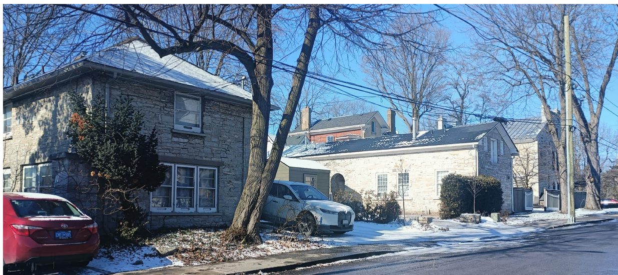
Figure 6: Maitland Streetscape looking northwest with new shed visible but set back from adjacent stone outbuildings. (Heritage Studio, February 2024)
