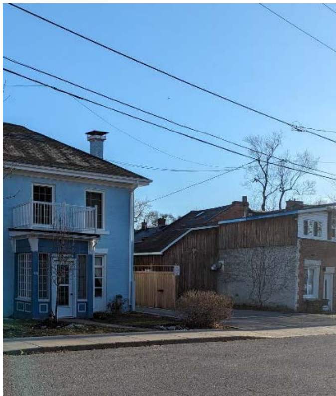
Above: Looking towards the rear of 160 Bagot Street from Lily Lane on Earl Street.
