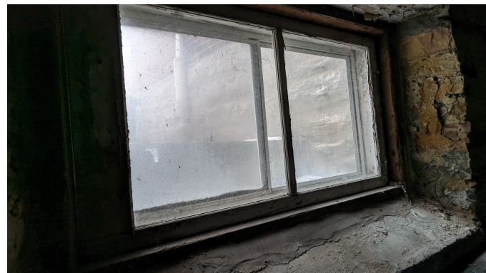
WINDOW 9 BASEMENT SOUTH
