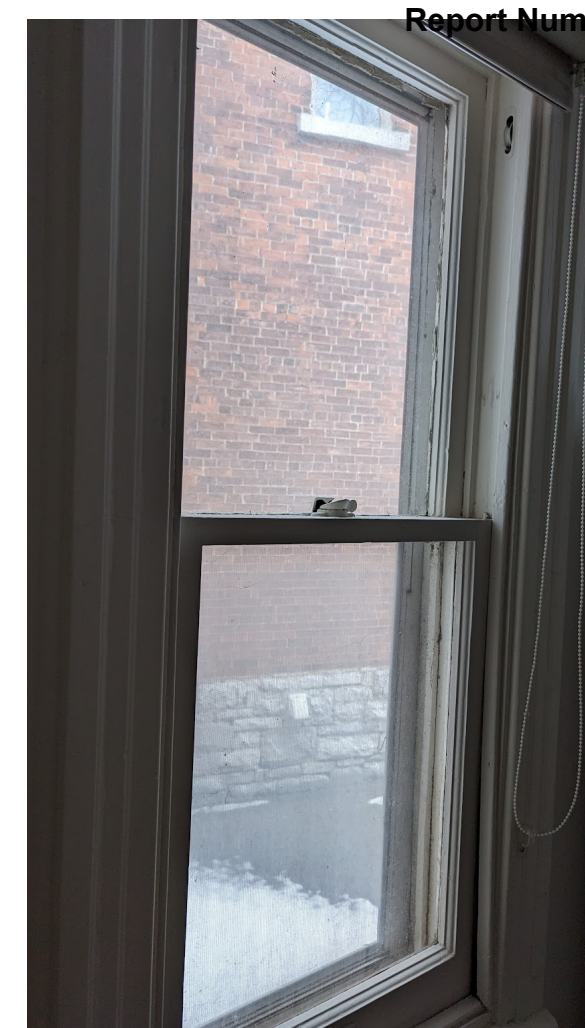
WINDOW 3 MAIN FL EAST
