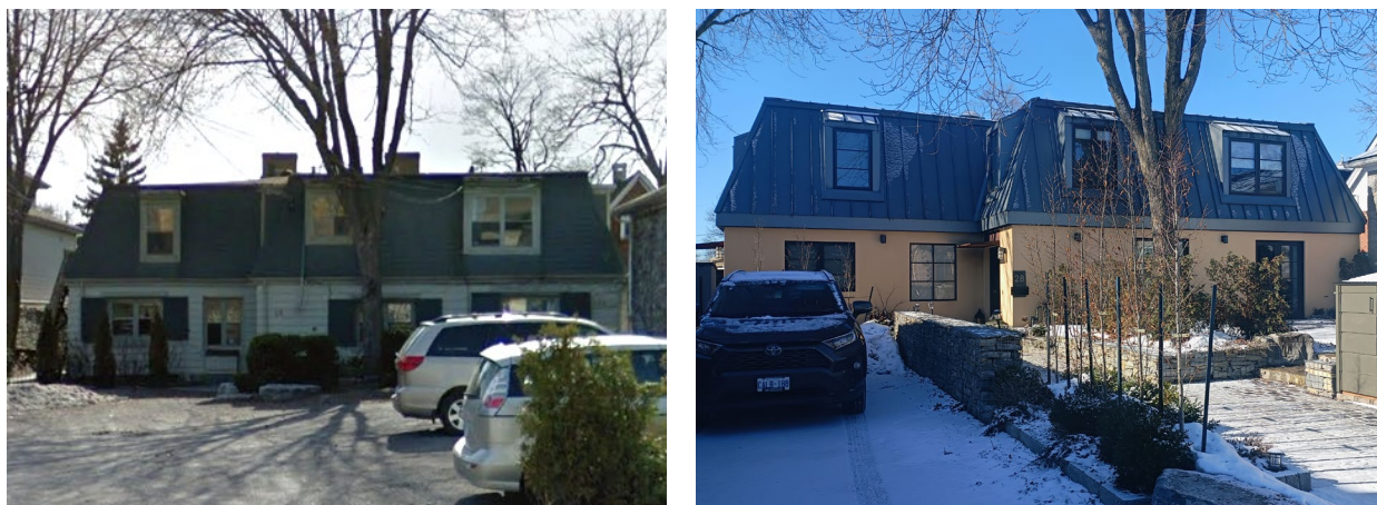
Figure 5: The subject property before and after rehabilitation to two separate residential units. (Google Maps and Heritage Studio, February 2024)
