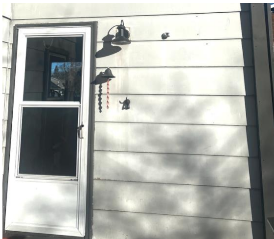
Addition back door and space for windows.
