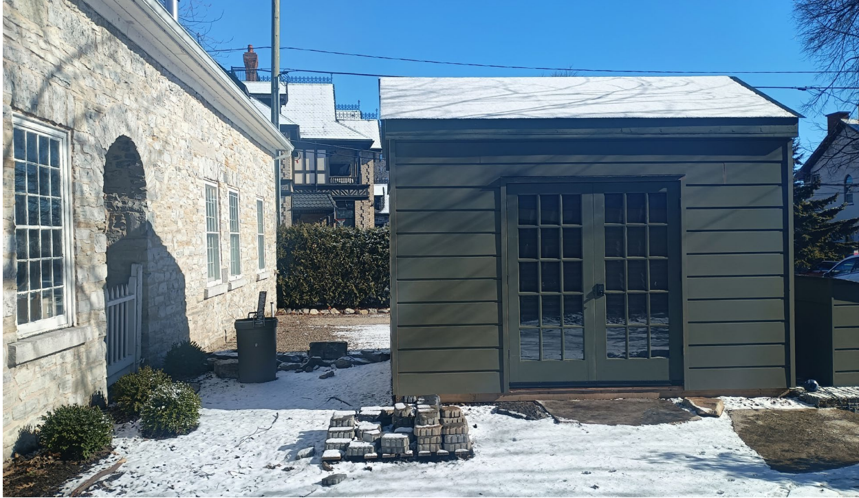
Figure 9: West elevation (facing the house) of the newly constructed shed. (Heritage Studio, February 2024)
