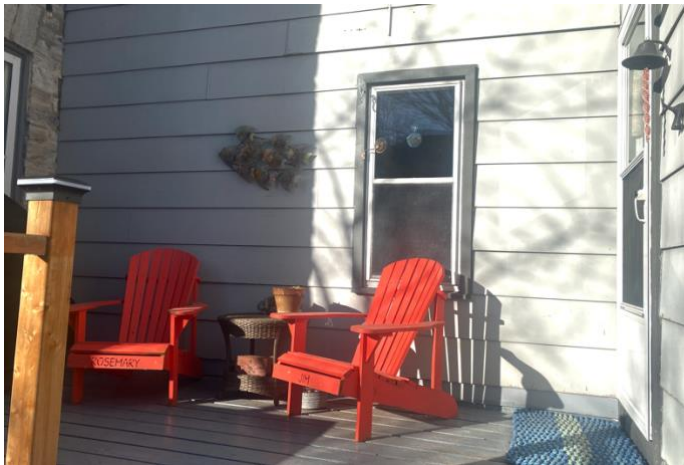
Existing kitchen east facing wall where door will be located.
