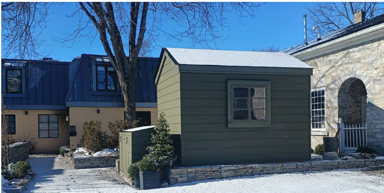
Figure 8: East and south elevations of the newly constructed shed. (Heritage Studio, February 2024)
