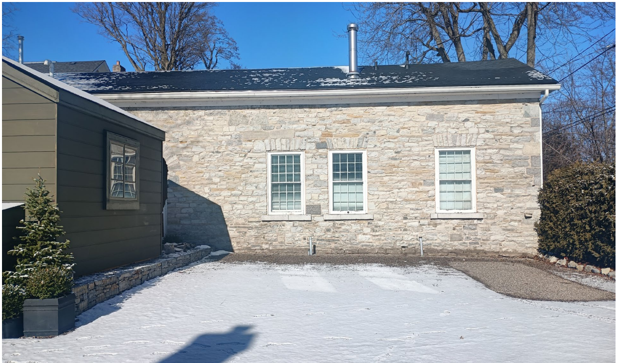
Looking north towards the east elevation of the shed and the south elevation of the adjacent stone outbuilding.
