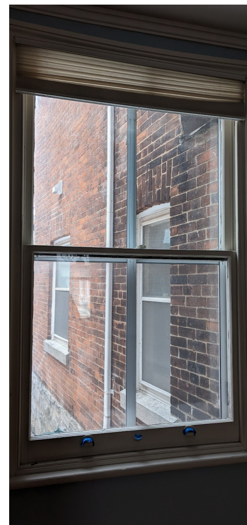
WINDOW 2 MAIN FL SOUTH
