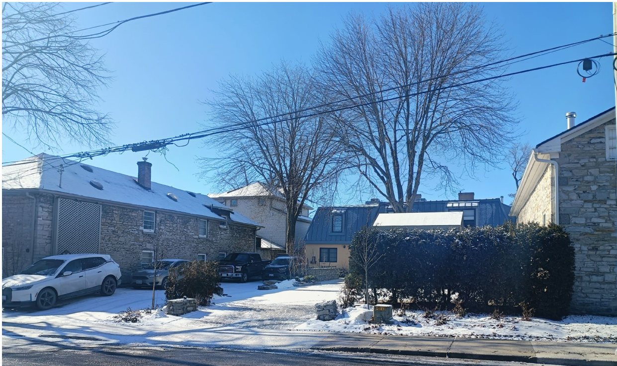
Looking west towards the property with shed and house behind, and two large stone outbuildings flanking the property.
