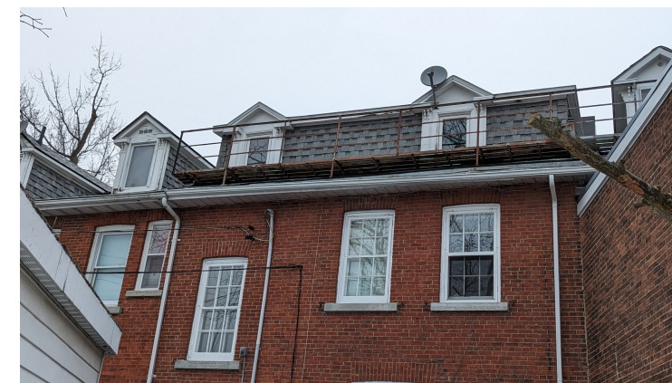
SOUTH SHED DORMER at 160 EARL
