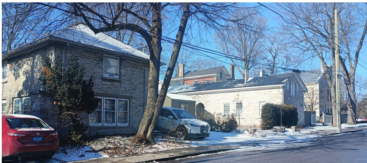
Figure 6: Maitland Streetscape looking northwest with new shed visible but set back from adjacent stone outbuildings. (Heritage Studio, February 2024)
