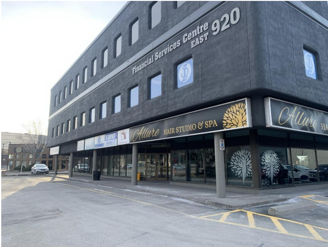
Figure 6. The existing building addressed as 920 Princess Street on the subject property, which includes a variety of commercial opportunities (photo taken March 22, 2024).
