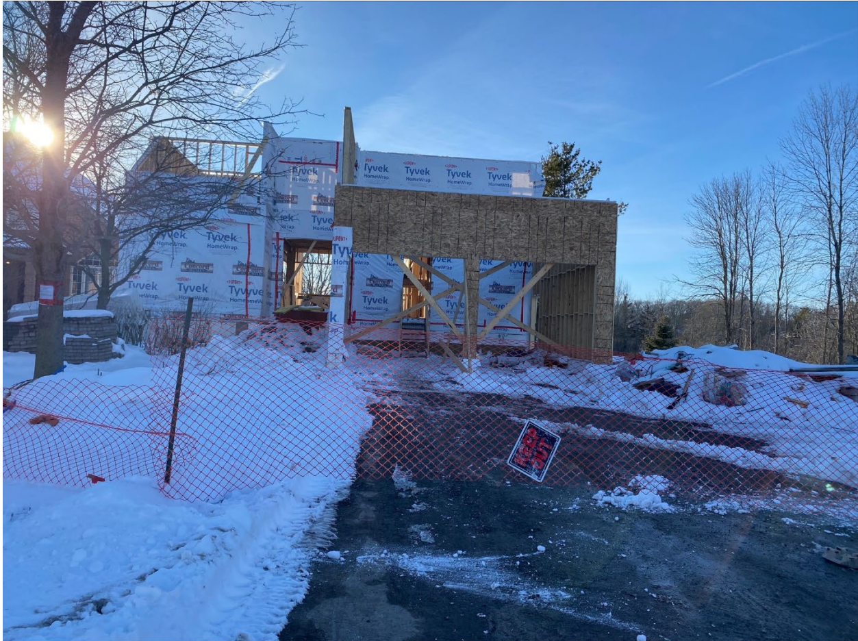
Figure 2: The neighbouring property, 927 Malvern Terrace, was destroyed by fire in January 2022, and is now being re-built. For contextual purposes, it is a two-storey home of a similar size to what is proposed at 931 Malvern Terrace, which would be situated on the right side of the image.
