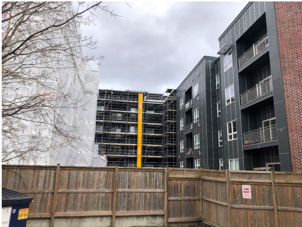
Figure 4: Rear interior courtyard.
