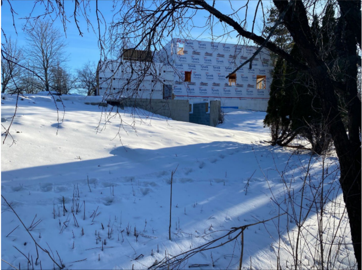
Figure 5: The subject site, viewed from the edge of the Open Space area, looking south. The foundation of the former home is visible towards the centre of the image, with the new home currently under construction at the neighbouring property visible beyond.
