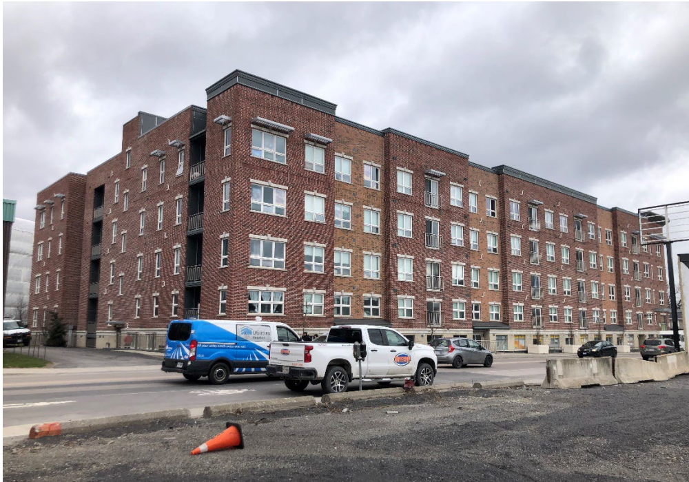
Figure 1: Princess Street (south) and side (west) elevations.
