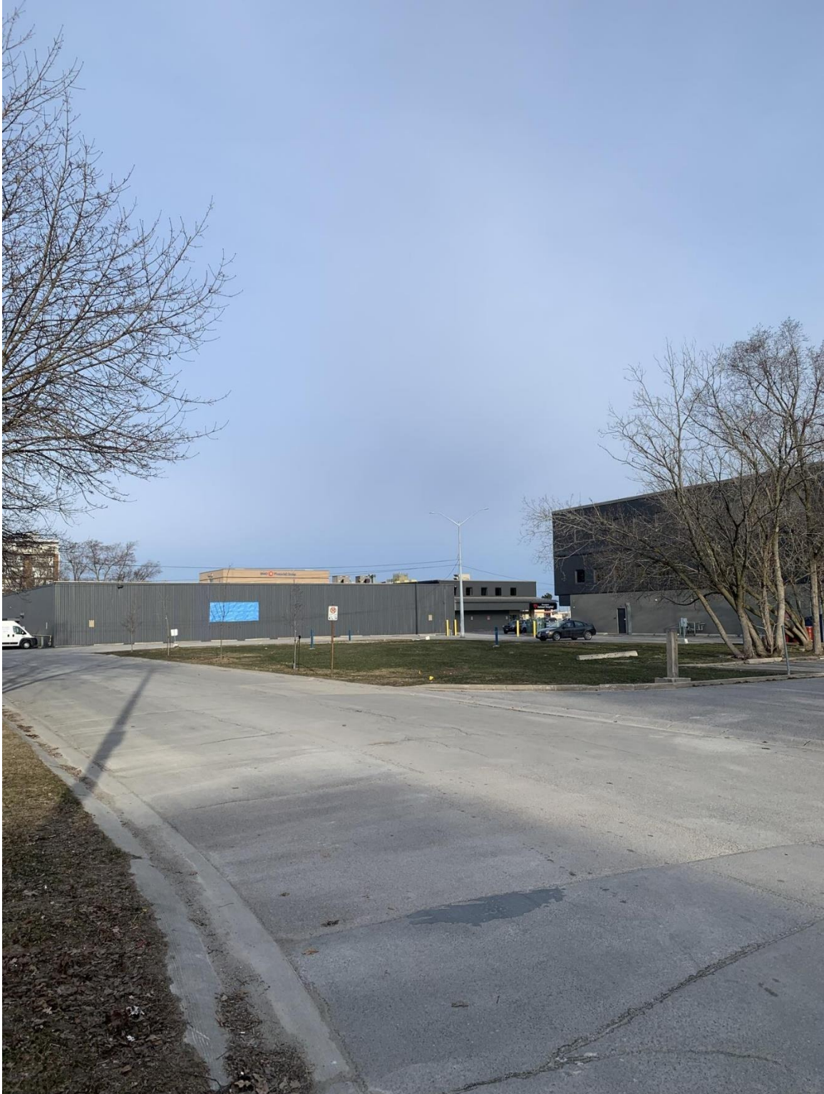
Figure 12. West facing view along Franklin Place towards the vacant portion of the subject property (photo taken March 22, 2024).
