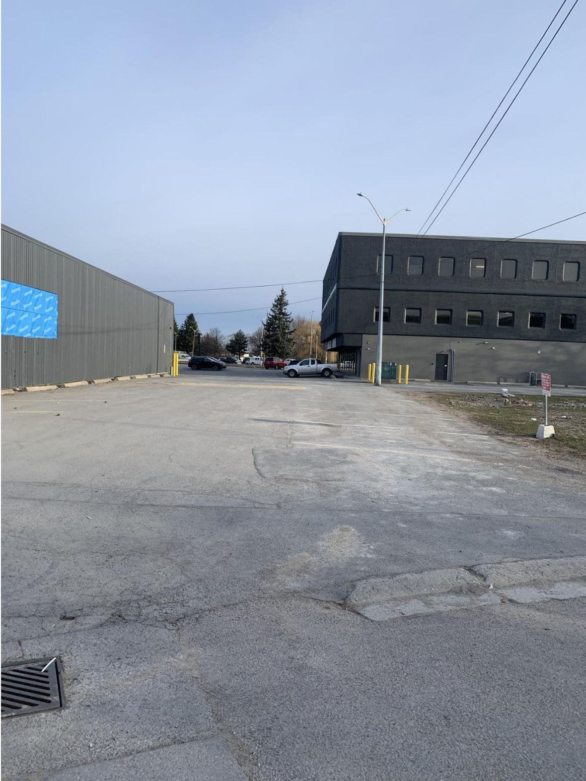
Figure 3. North facing view along the Franklin Place frontage of the subject property demonstrating the existing paved parking areas (photo taken March 22, 2024).
