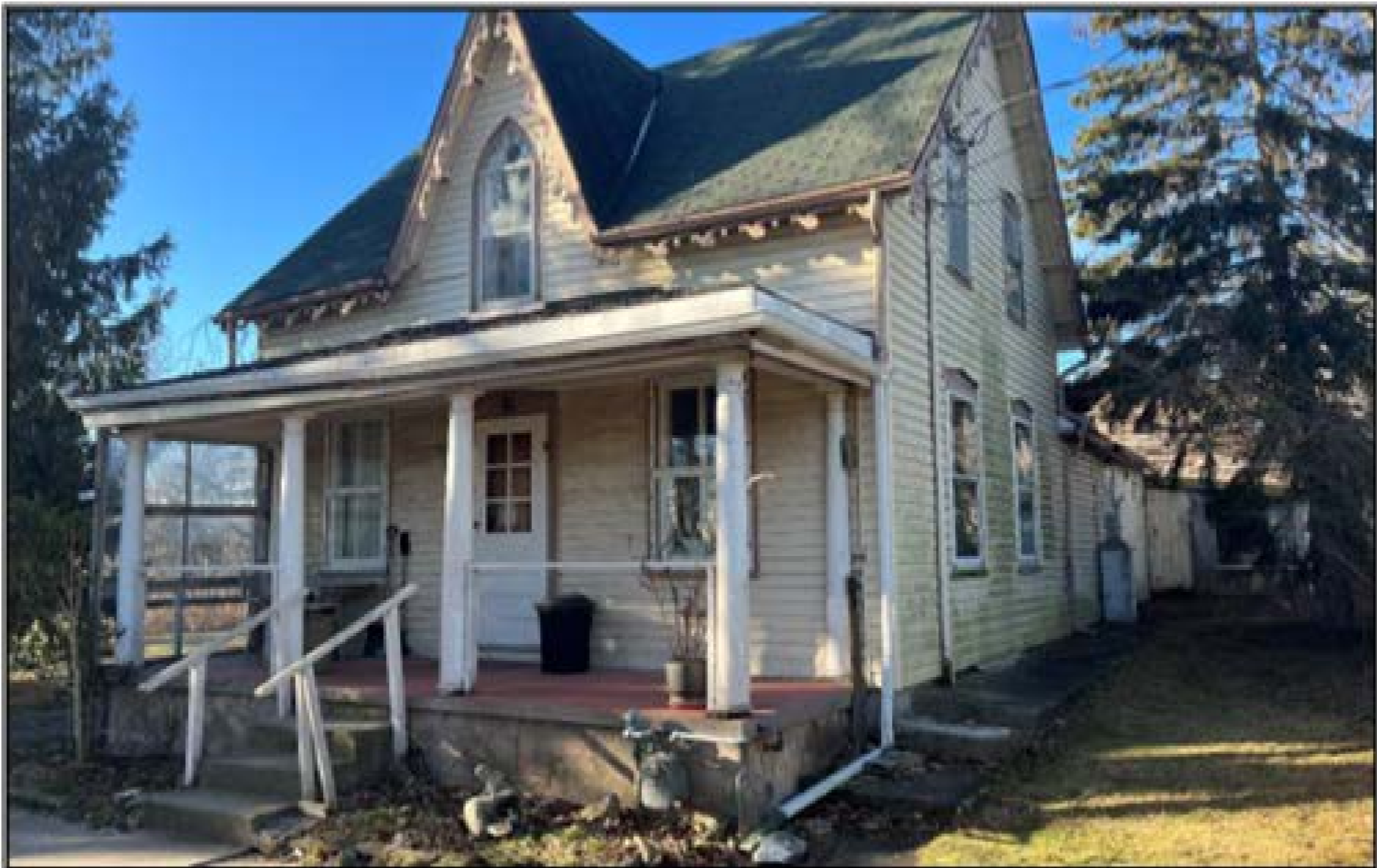
Front view of the subject house looking south-westerly
