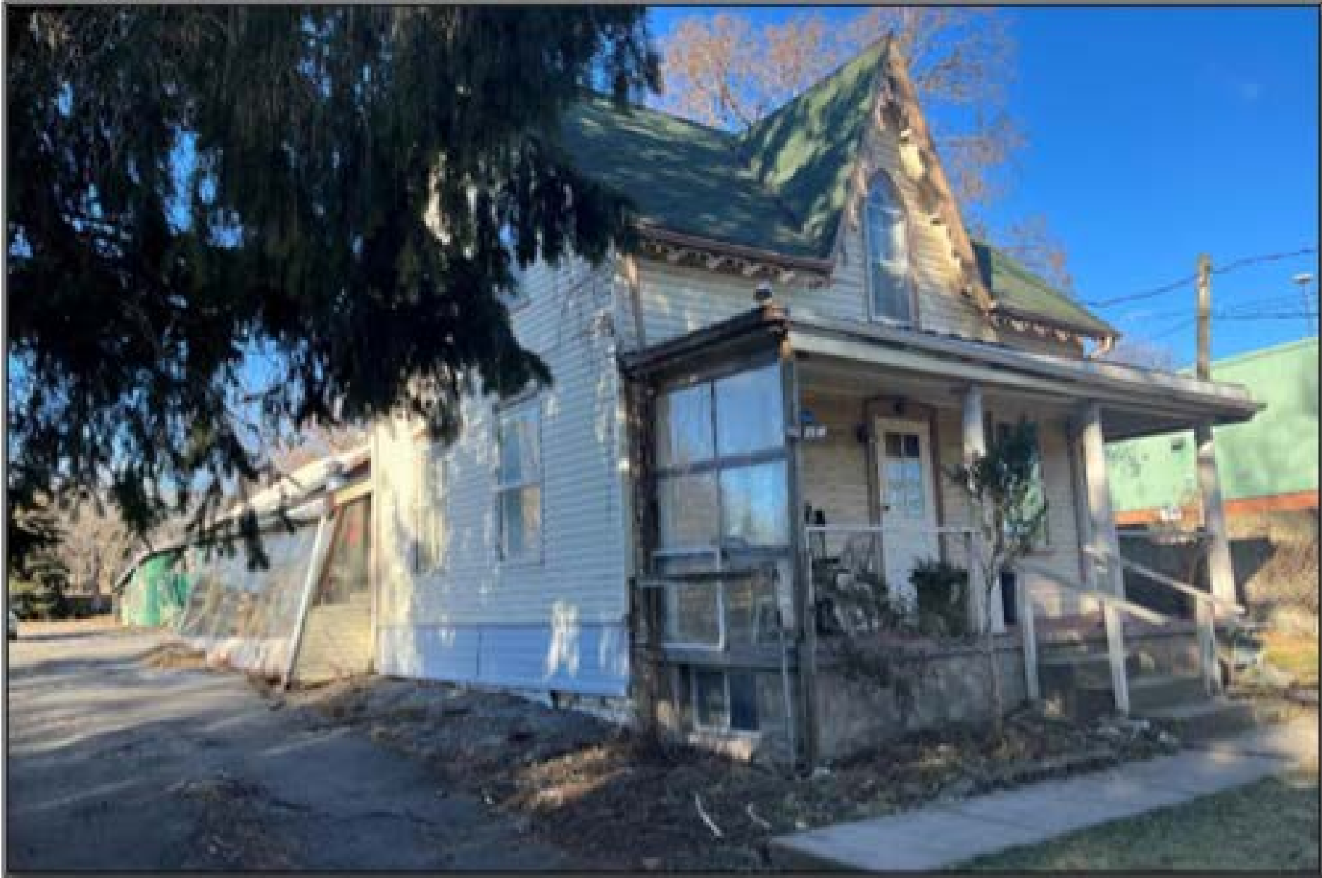
Front view of the subject house looking north-westerly
