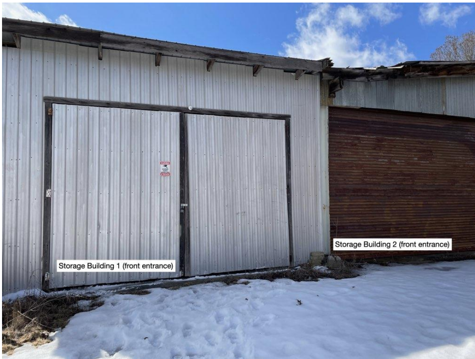
Figure 4: Storage building on the retained parcel associated with the existing workshop use.
