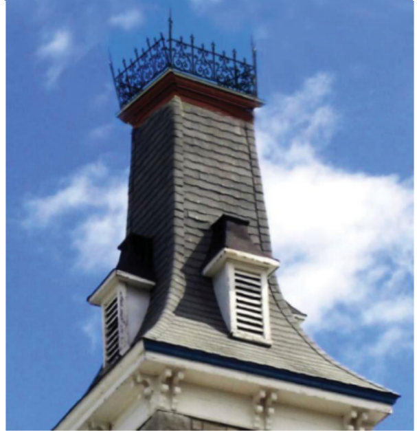
See the Hewett House of 1875 RMC, for a recently replaced metal fringe
