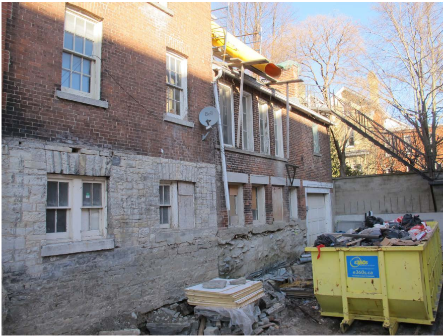
Subgrade conditions on hotel and courtyard
