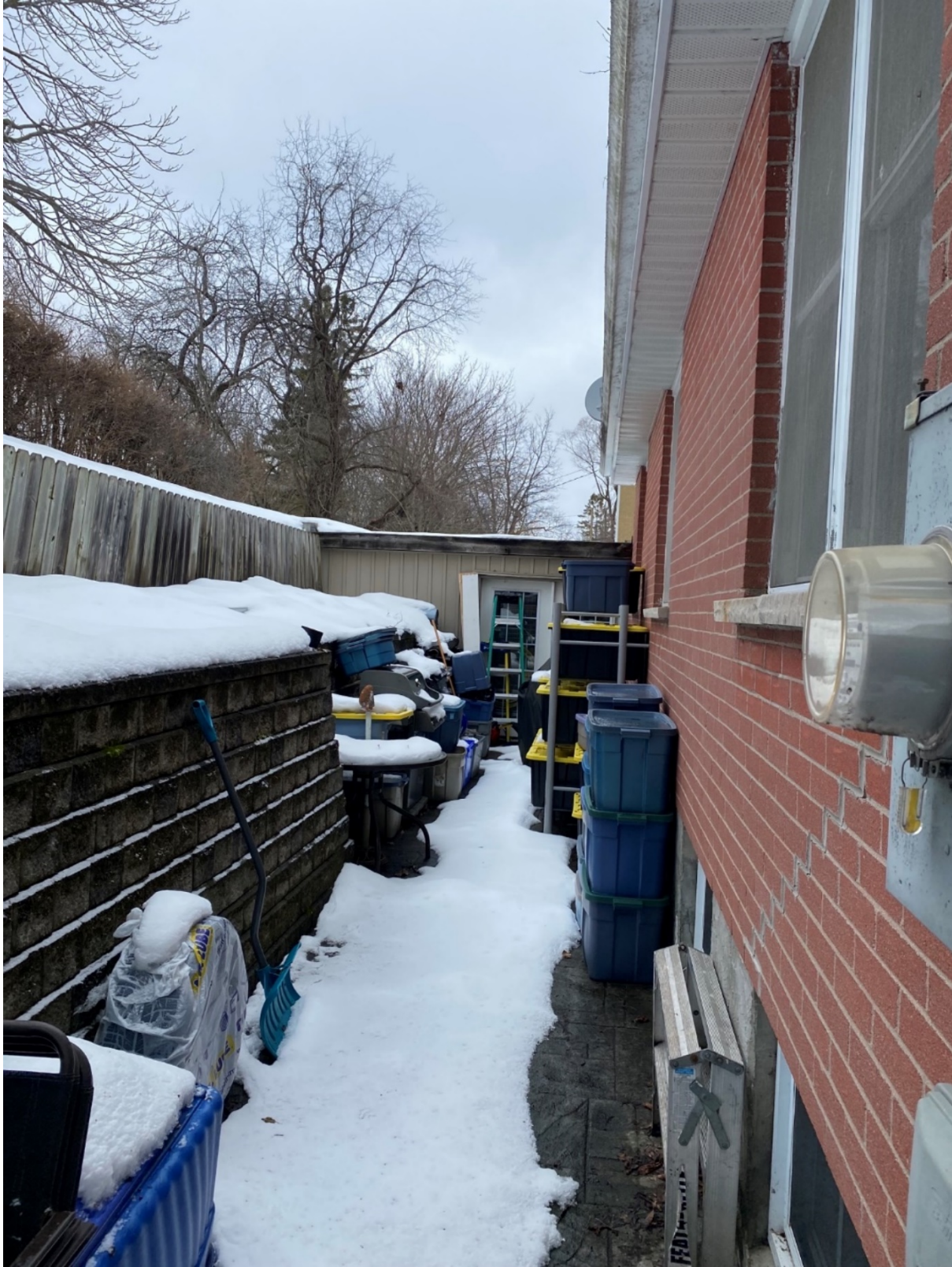
Rear yard of the subject site with the retaining wall to the left. The current garage will be removed.
