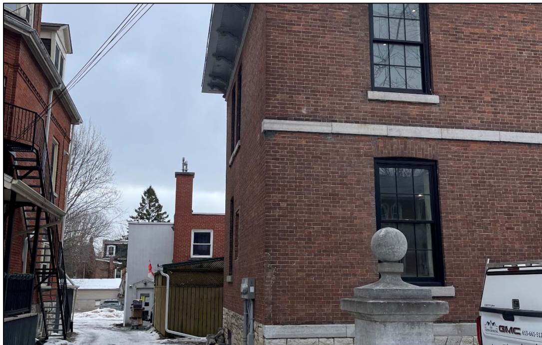
Figure 2: View of rear lane from Bagot Street
