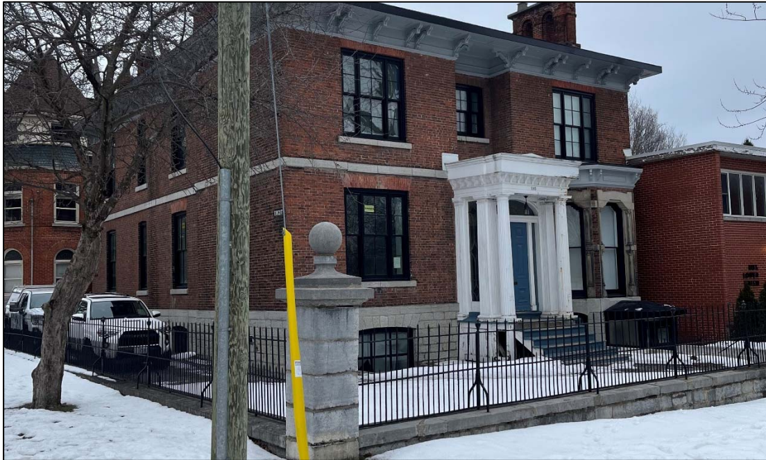
Figure 1: View of the Subject Property from the Corner of Bagot St and Lower Union St
