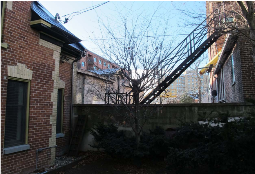
View west from No. 155 King Street East
