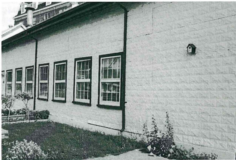
Figure 7: Detail of c1915 addition.
