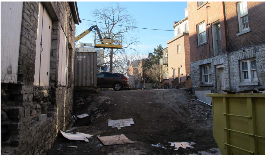
View west of rear of No. 131-33 King Street East
