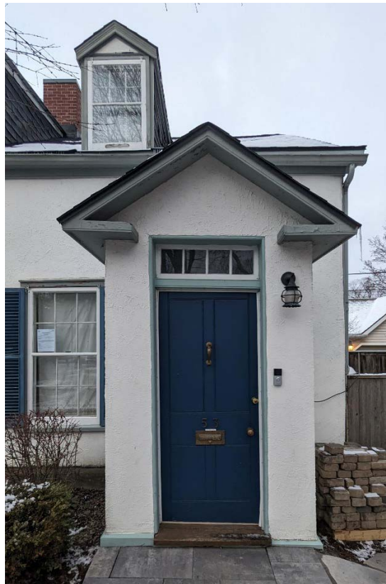
Below: Entryway vestibule head on.
