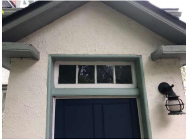
The above photographs show the soffit pulling away from the main structure. The transom is out of level in relation to the front door. Both cases likely due to structural settling.
