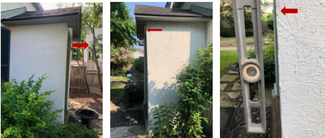
The images above show the street-facing wall four inches out of plumb. Its top leans toward the street. This is likely due to lack of a proper foundation.
