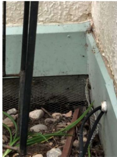
Finally, the above photographs document a lack of perimeter foundation. Soil is up into the floor plenum.
