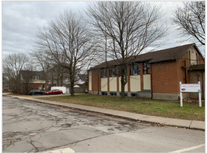
Looking south across Earl Street opposite the subject property
