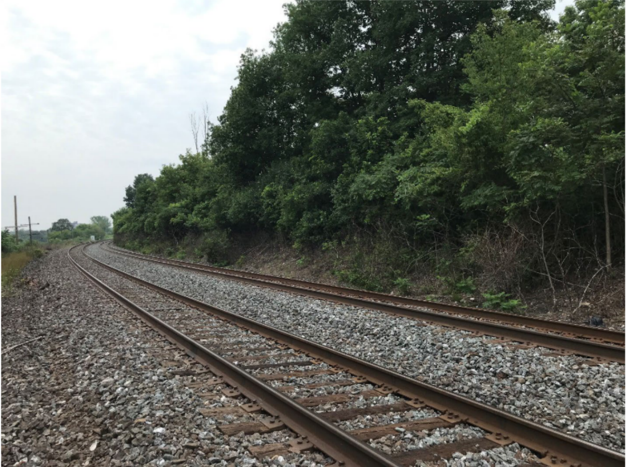
Figure 5: The CN rail line, looking south, abuts the eastern boundary of the site, pictured here to the right. The development will be set back 30 metres from the rail corridor, within which a treed berm is proposed for enhanced safety measures, along with the already significant grade change between the property and the railway.
