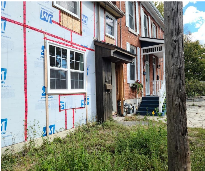
Figure 2: North-east facing view of the front entrance. The proposed porch at 5 York Street would project outwards a similar distance to the existing porch in front of the adjacent rowhouses 3 York Street and 1 York Street.
