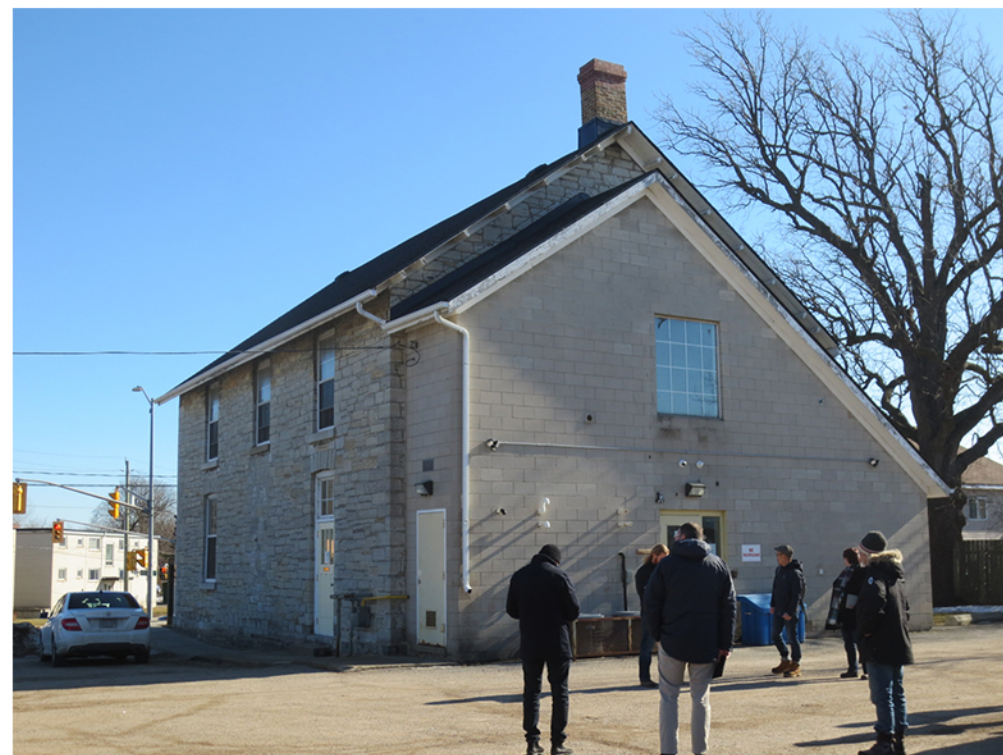
Existing addition exterior
