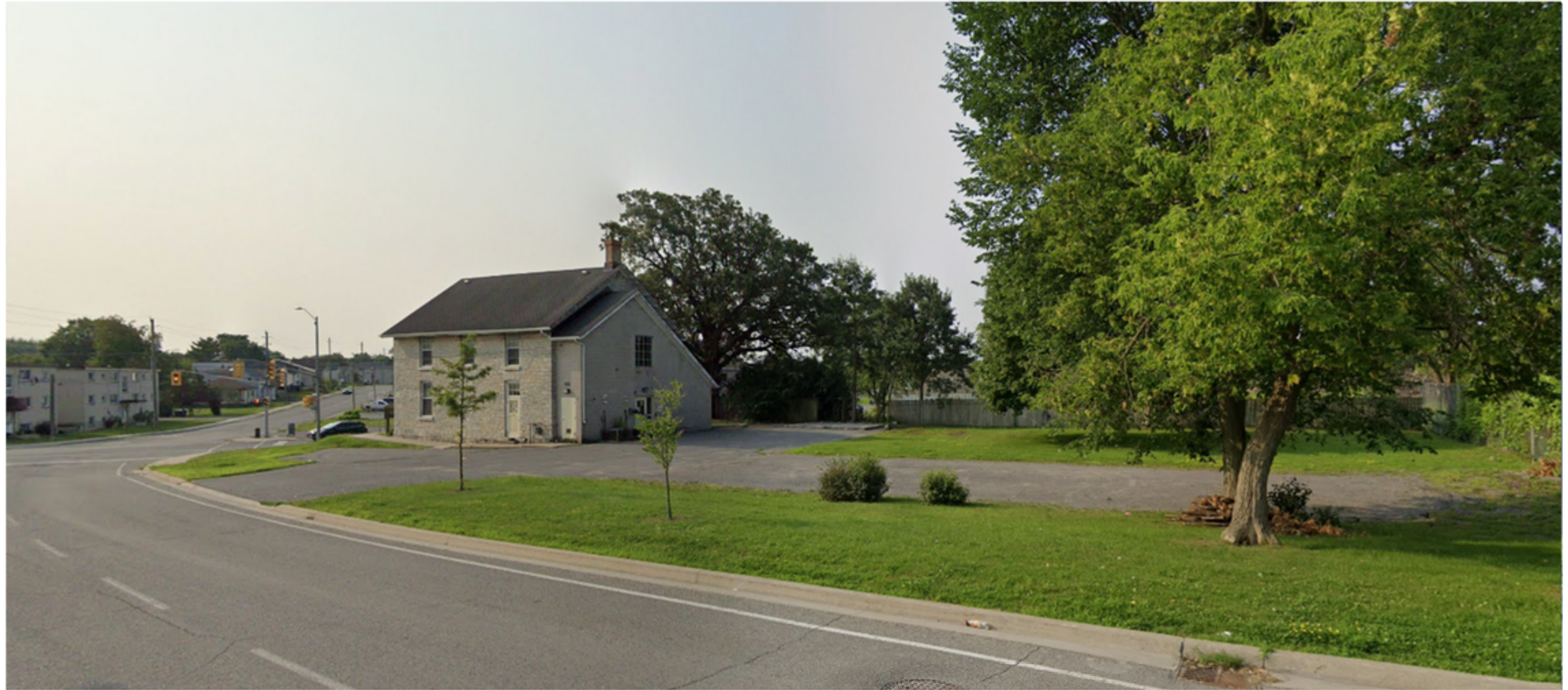
Existing heritage building with addition, and parking lot on site. View from Railway Street looking South-East
