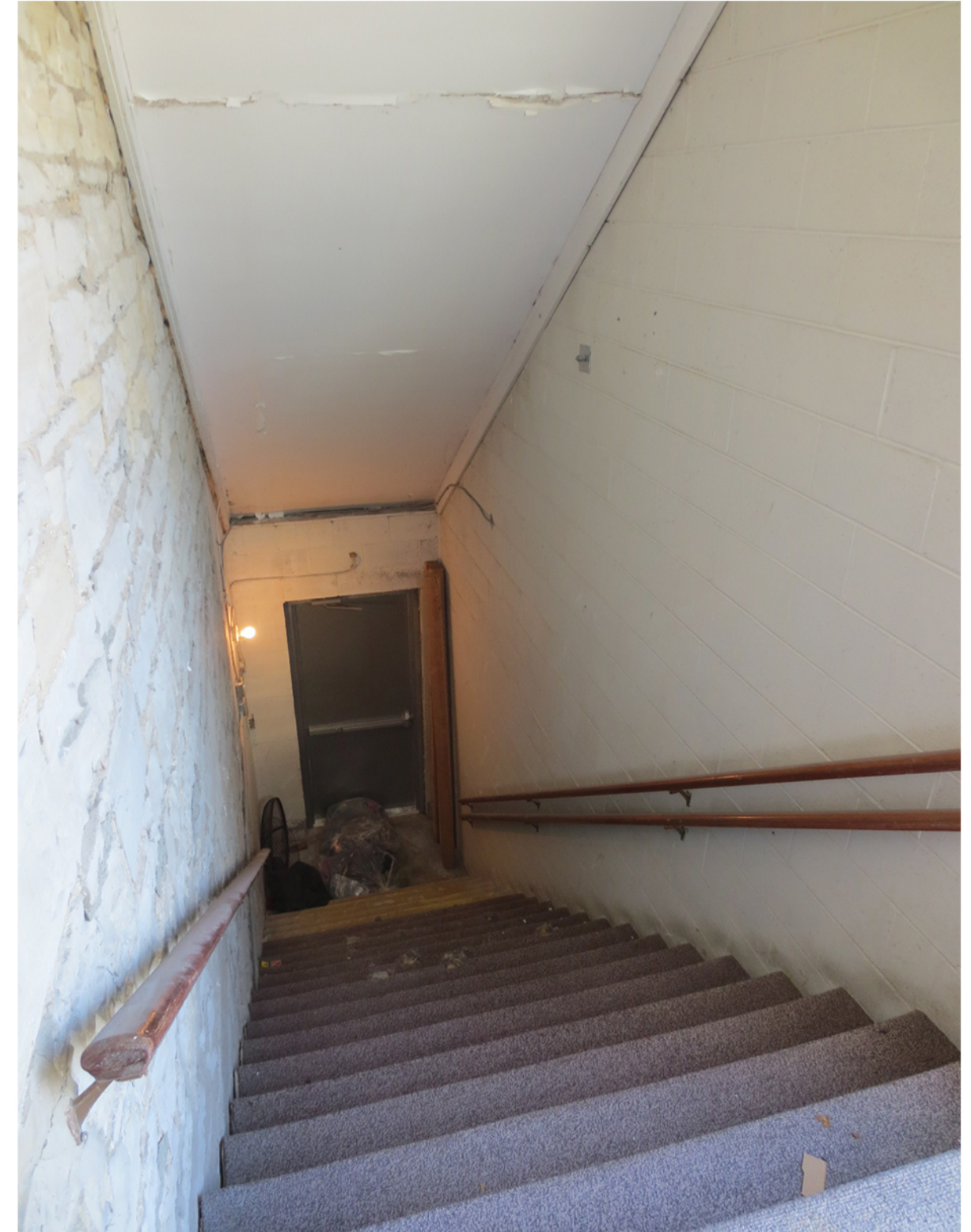
Existing addition interior
