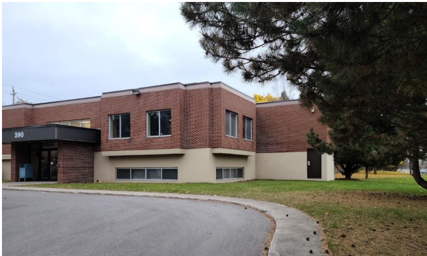
Figure 2: View of the north-east corner of the office building. A 211 square metre addition is proposed for the east side of the building.
