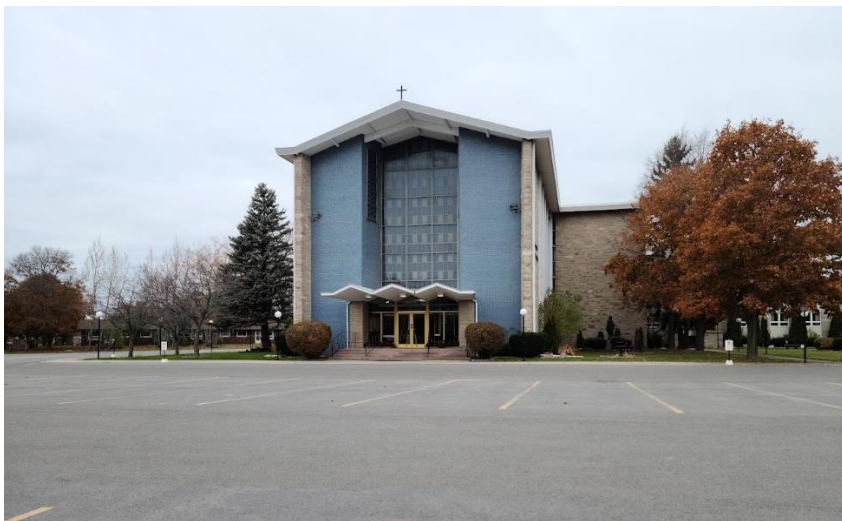
Figure 6: Frontal view of St. Joseph's Church, across the parking lot from the office building at 390 Palace Road.
