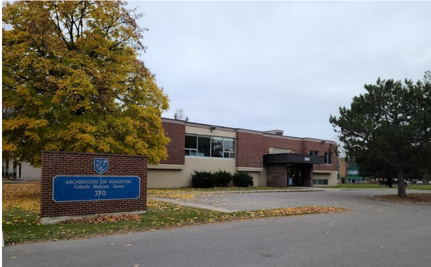
Figure 1: Frontal view of the office building at 390 Palace Road, known as the Francis J. Spence Pastoral Centre.
