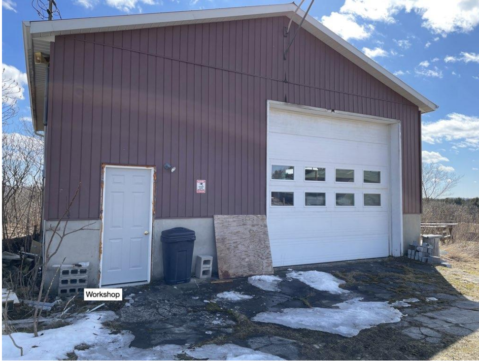
Figure 5: Exterior of the existing workshop building on the retained parcel. The workshop building is used for the repair of furniture and other similar items.
