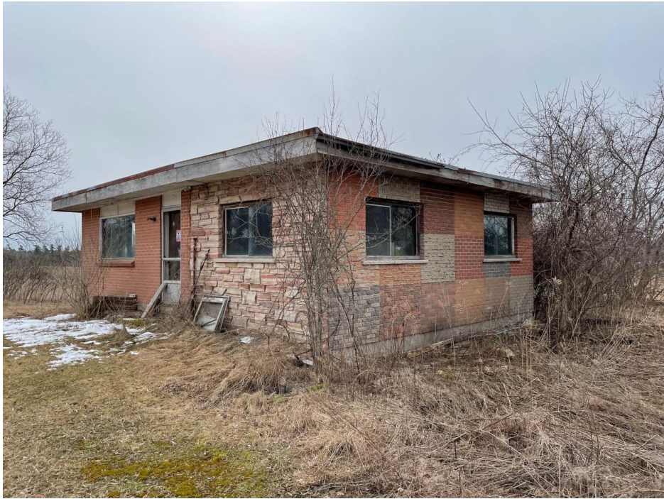
Figure 3: Former office building on the retained parcel of the subject lands, which was approved for conversion to an Additional Residential Unit through Permission application D13-015-2023.
