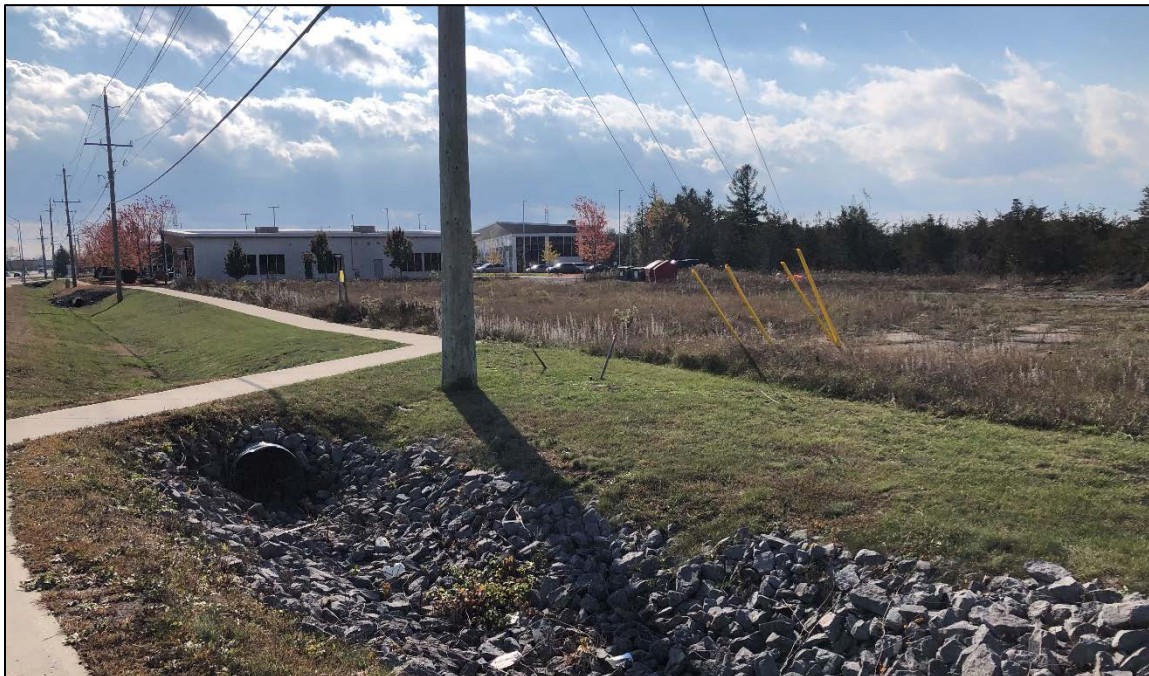
Figure 4: Street view of 1383 Gardiners Road (Location of Future Building A).
